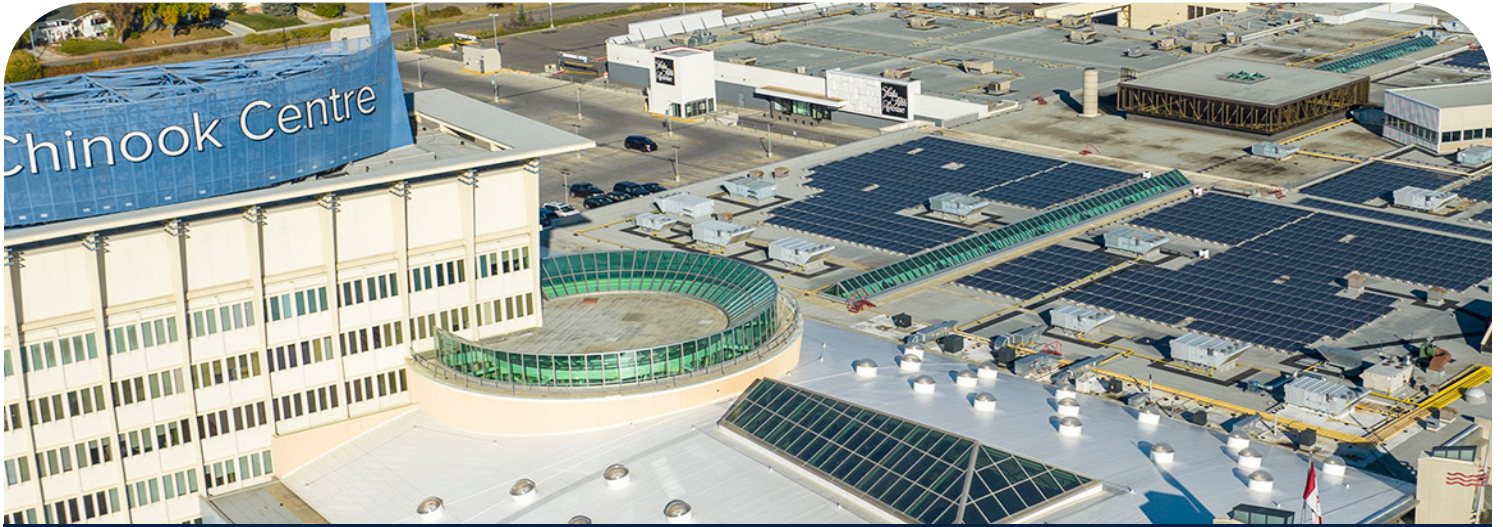
ENMAX Power solar panels, CF Chinook Centre (Calgary, Alberta)
