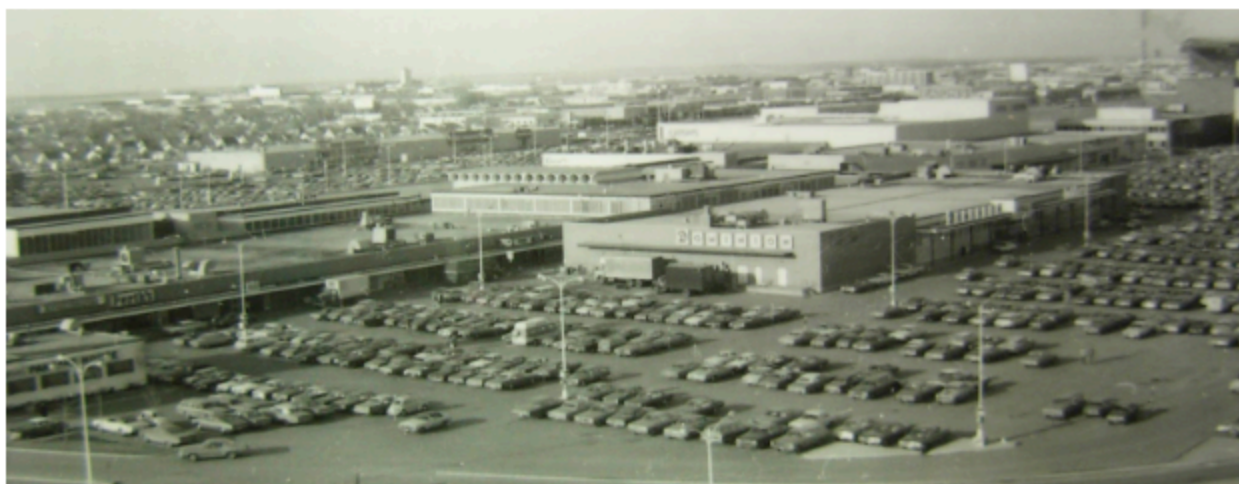
Completed Dominion and Loblaws stores in the east wing expansion. 1974 - Archives of Manitoba, CH 0267 Government photographs.
