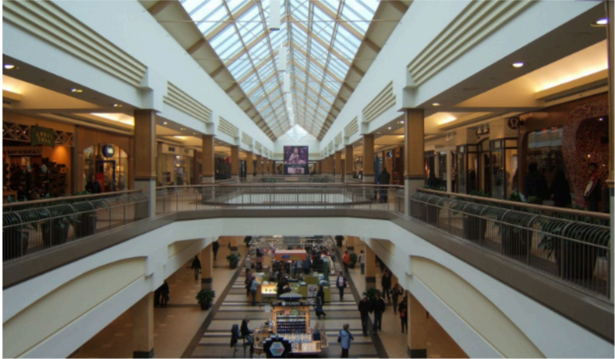
The redesigned interior in 2007 during the later phases of construction. Photo from CF Polo Park archives.
