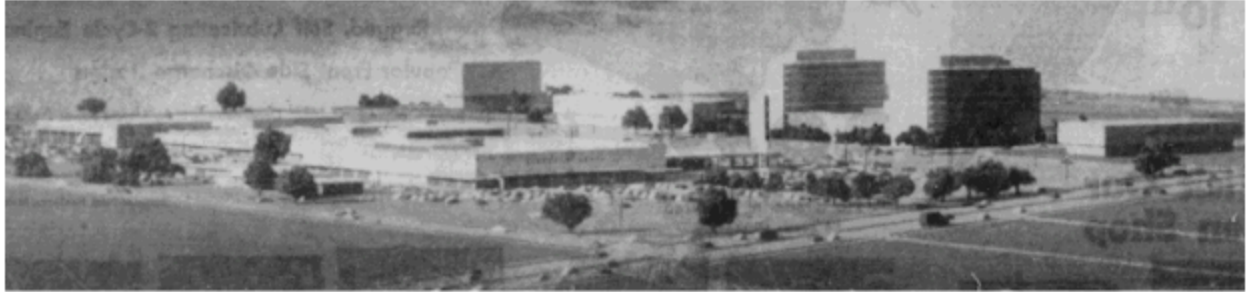
Scale model of the proposed shopping centre and surrounding development Winnipeg Tribune, May 5 1959
