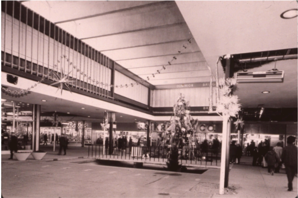
Centre court during the holidays in 1963. Roof construction was still ongoing. From Vintage Winnipeg.
