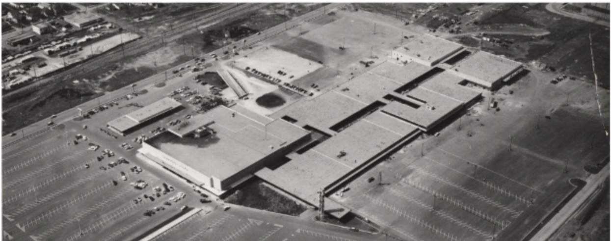
Polo Park Shopping Centre during final stages of construction in 1959 Here, Simpsons-Sears had already opened prior to the remainder of the mall being finished. Photo from CF Polo Park archives
