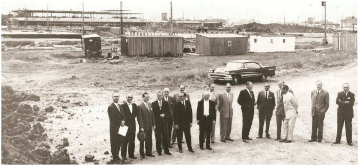
Polo Park in the initial stages of construction. From CF Polo Park archives
