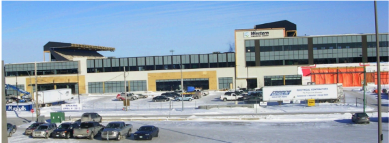
Polo North under construction, 2013. Photo from CF Polo Park archives.
